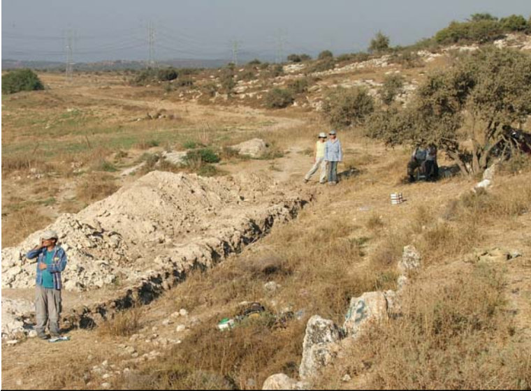
Figure 6: View, generally looking East, of dug ground-truth trench. Area is located just north of GPR 2004 Grid Area 1.
